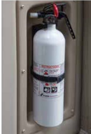
Typical Class B-C fire extinguisher
