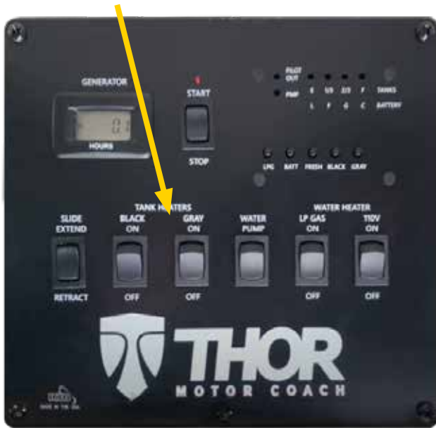
Holding Tank Heater Control Switches
