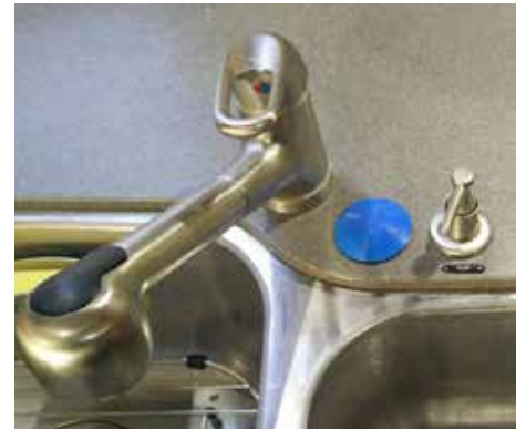
Example of an installed Sink Miser. Note the blue indicator button (mushroom).
