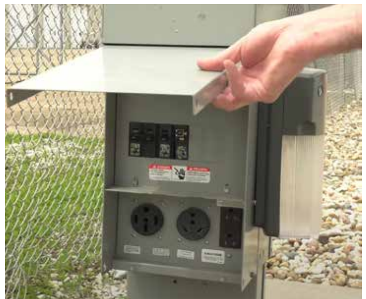
Typical Campground electrical service stand. This illustration shows 50 amp, 30 amp, and 15-20 amp outlets, along with corresponding circuit breakers.
