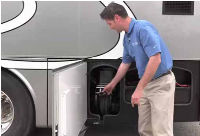
50 amp shore power cord attached to an electrical-powered reel.
