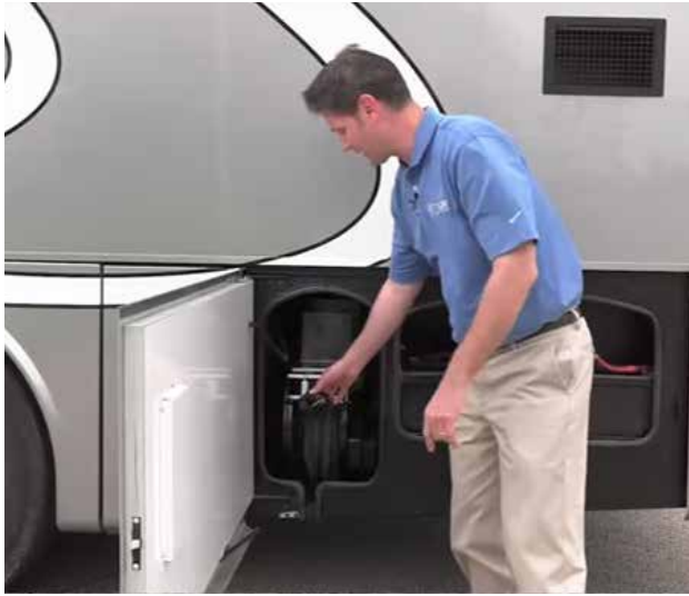
50 amp shore power cord attached to an electrical-powered reel.
